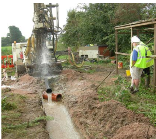
Plate 7 Water being air flushed from the La Rocque borehole at the rate of 7 l/sec (607 m 3 /d) from 43 m bgl, prior to the setting of casing and grout to that depth.
