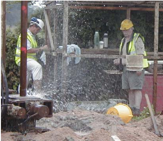
Plate 4 Monitoring penetration rates.
