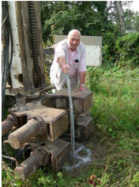
Plate 1 and Plate 2 Accurate positioning of the drilling rig.
