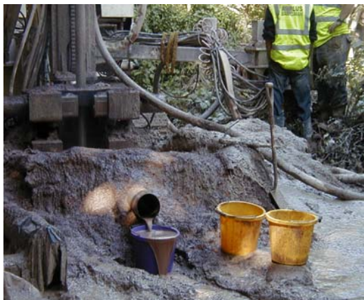
Plate 10 Muddy water discharging from St Catherine borehole at about 0.27 l/sec (23 \text{m}^3/\text{d} ) from 75 m bgl.
