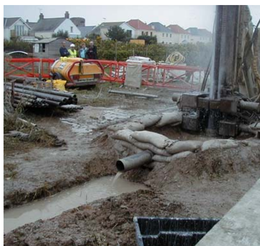
Plate 7 Water being air flushed from the La Rocque borehole at the rate of 7 l/sec (607 m 3 /d) from 43 m bgl, prior to the setting of casing and grout to that depth.
