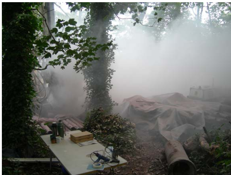
Plate 9 Excessive quantities of rock dust blown from the St Catherine borehole during drilling at 33 m bgl.
